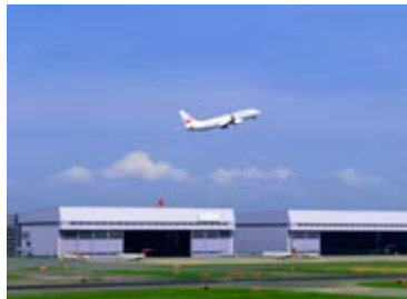
IIF Haneda Airport Maintenance Center
