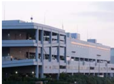
IIF Shinonome Logistics Center
