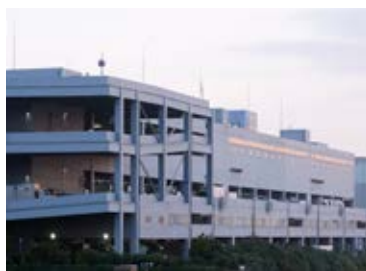
IIF Shinonome Logistics Center
