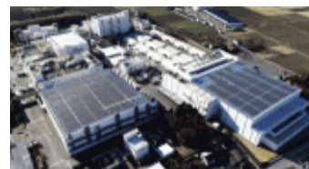
Photovoltaic power generation has been introduced in the Kao Tochigi Plant to provide the power used by the plant
