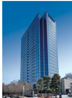
1-minute walk from JR and Tokyu Musashi-Kosugi Station, a large office building with high visibility from the station
