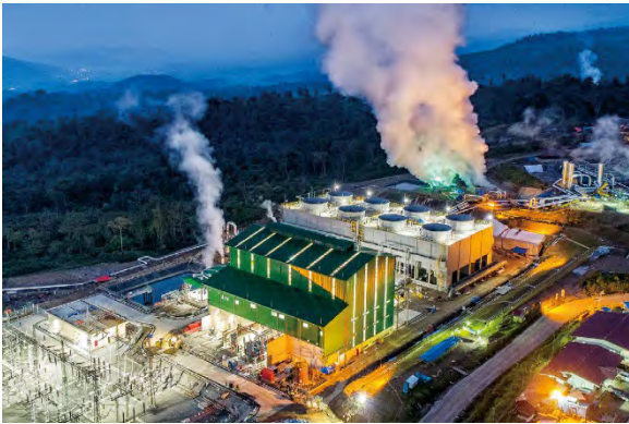
Muara Laboh Geothermal Power Plant
