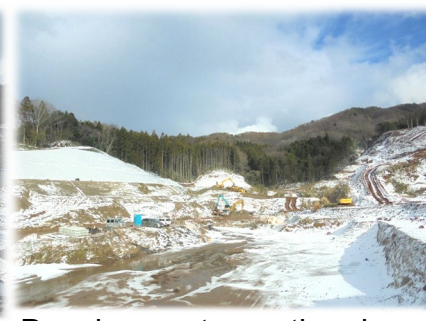
Development near the phase 1 landfill site
