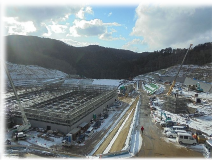
Area surrounding the leachate treatment facility
