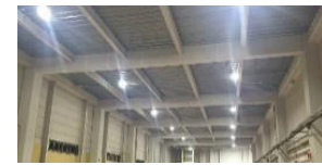
Installing LED based on green lease agreements
