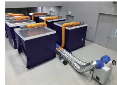
Full view of the anti-COVID-19 air-conditioning and ventilating booth for anti-disaster shelters
