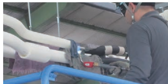
Aluminum pipes brazing work
