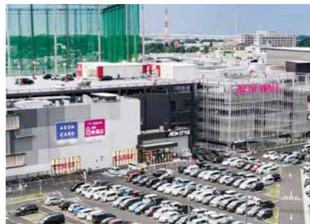
Aeon Mall Kawaguchi, an effectively net-zero CO 2 emissions mall for power supply and gas
