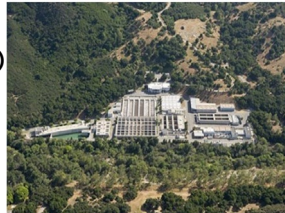
Tapia Water Reclamation Facility (California, USA) (Photo credit: Las Virgenes Municipal Water District)
