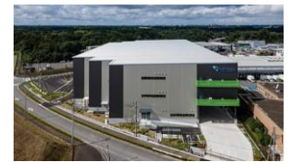
Odakyu Real Estate Inzai Logistics Center
