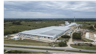
New float furnace in Argentina
