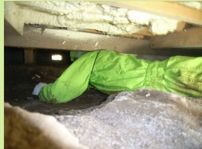
<Working under the real floor>
