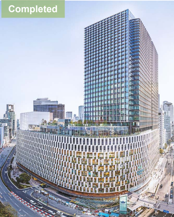
Osaka Umeda Twin Towers South (Osaka, Japan) Total of 23, 17 elevators and 6 escalators
