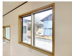
Example of installing double-paned window
