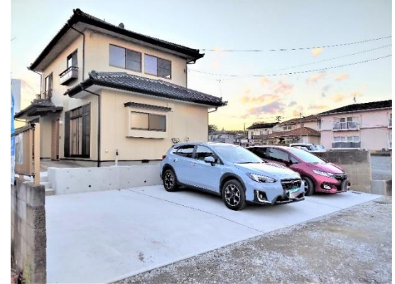
Removed the gate and front yard to create four parallel parking spaces that can comfortably accommodate visitors.
