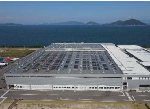
Solar power generating equipment on the roof of Kozai Plant
