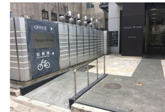
Barrier-free renovation construction (Tenjin Prime)
