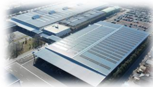
Solar Electric System (Ota Door Plant)
