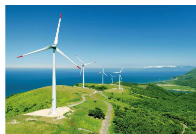
Shiribetsu Wind Power Plant (Hokkaido Prefecture)
