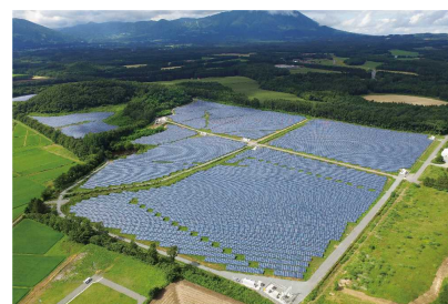
Shizukuishi Solar Power Plant (Iwate Prefecture)
