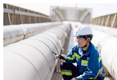
Bridge pipe safety inspection
