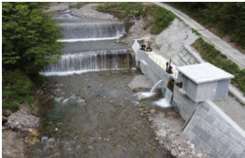
Small hydroelectric power plant: Aino-mata-dani Small Hydro Power Plant
