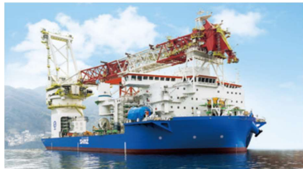
A Self-Elevating Platform (SEP) vessel under construction
