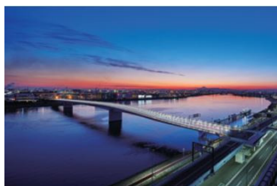
Illuminated Tamagawa Sky Bridge
