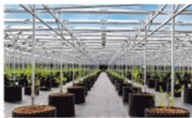
Tokorozawa Kitaiwaoka Solar Power Plant (solar sharing)
