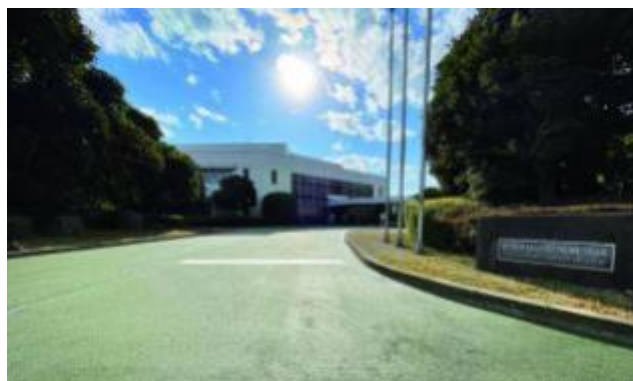
Experimental pavement of asphalt using synthetic calcium carbonate (carbonate) with immobilized CO2
