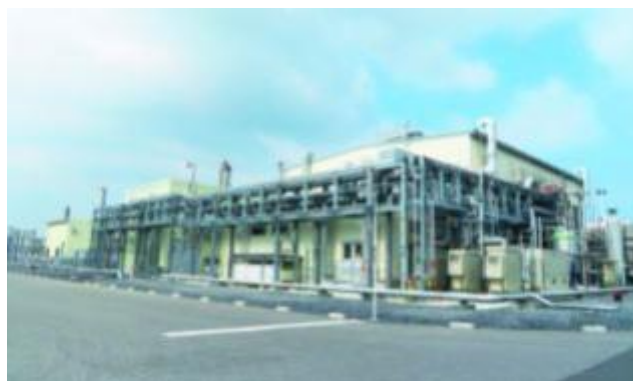
Demonstration facilities toward commercial production of solid electrolytes for next generation batteries
