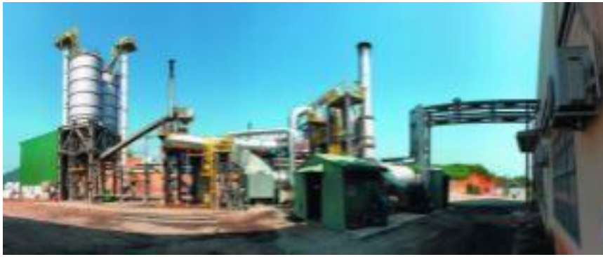
Demonstration plant for Idemitsu Green Energy Pellet
