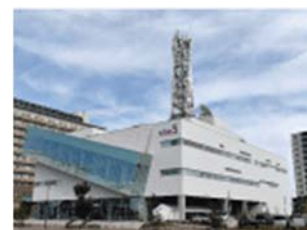
HIGASHI NIPPON BROADCASTING's new premise
