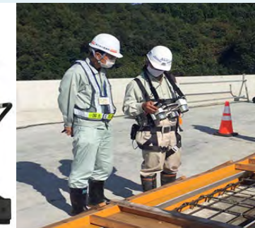
Inspecting rebar arrangement
