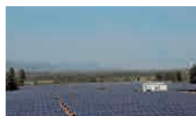
Vizag Plant's (India) power source
