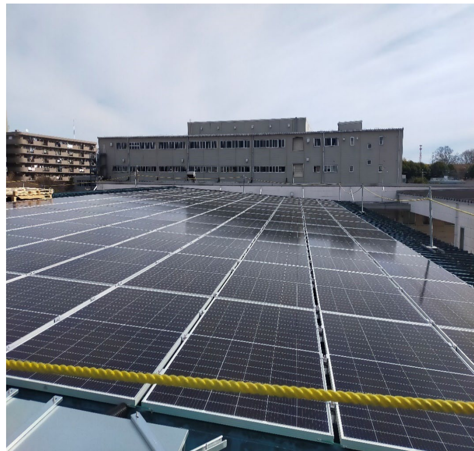
Kanto Factory in January 2022 Installation of solar panels
