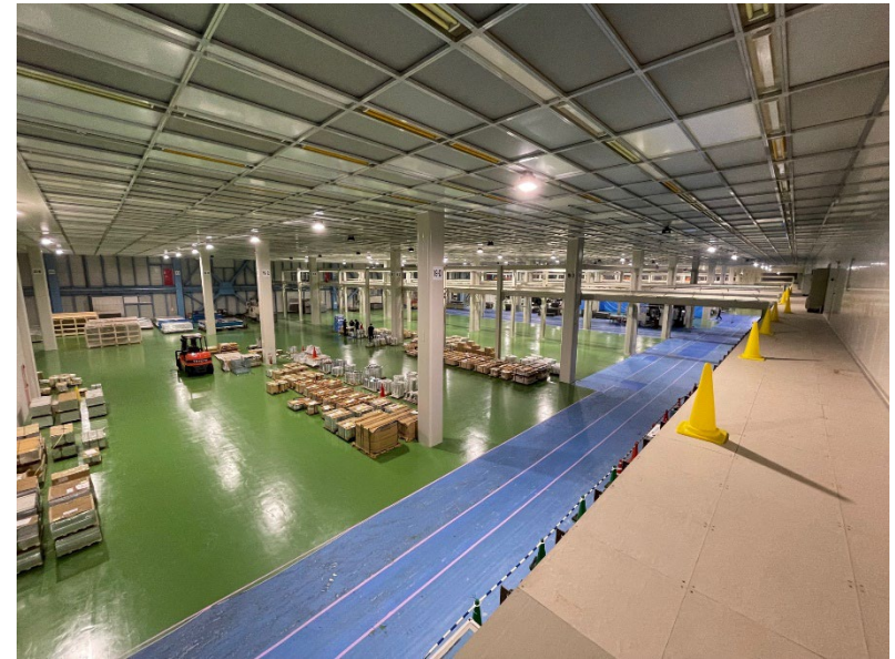
New expansion (under construction) Approx. 5,000 m 2
