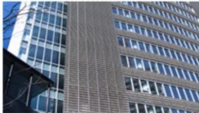
Introduction of renewable energy at our offices
