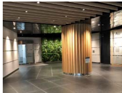
Renovation of entrance (Shin-Yokohama TECH Building)
