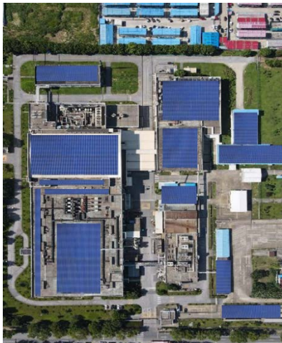
(Solar panels are dark blue.)
