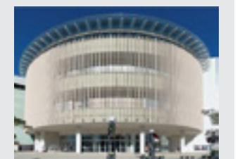
Solar power generation equipment
