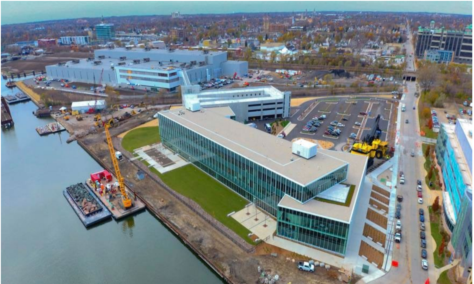
Komatsu Mining New Head Office Manufacturing Facility (South Harbor Campus)
