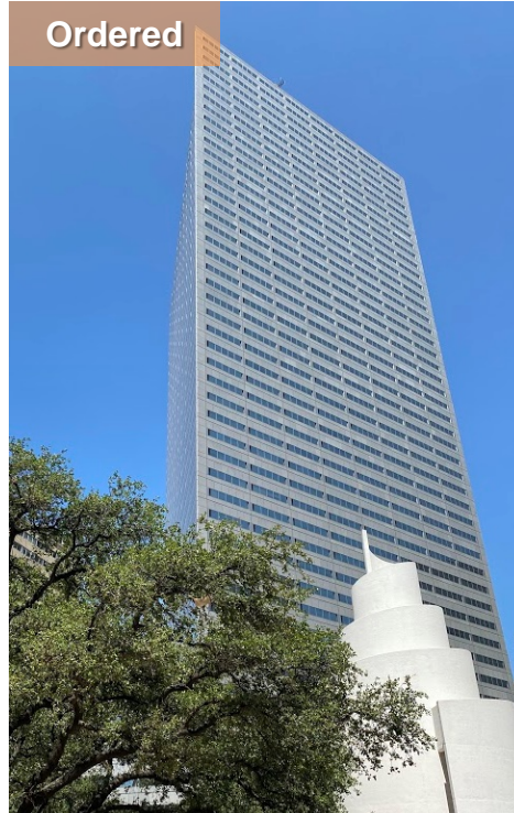
Energy Plaza (Dallas, USA) Total of 18 elevators
