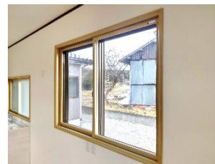
Example of installing double-paned window
