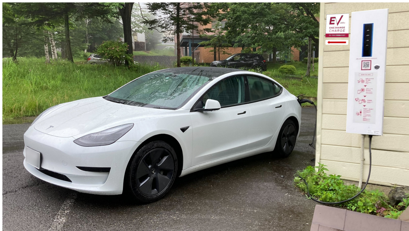
ENECHANGE EV Charging Service charging station installed at Kusatsu Onsen-ryokan Eidaya
