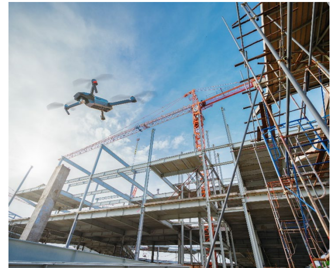
Mapping and surveying
