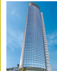
Nakanoshima Mitsui Bldg. (Osaka City, Osaka)
