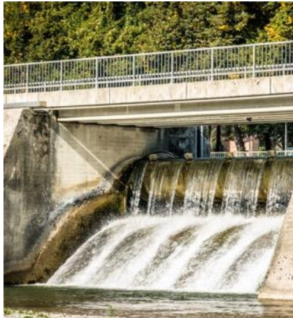
Small hydropower generation
