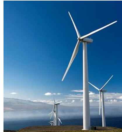
Wind power generation
