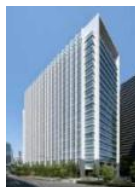
ARK Hills South Tower
