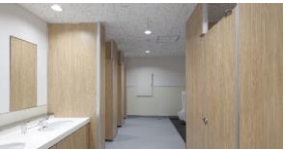
Installing water-saving toilet system
