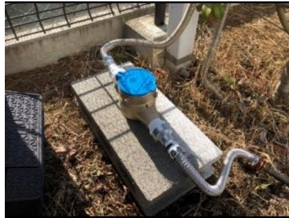
Install sub-meters on automatic sprinklers and monitor water consumption in more detail to save water
