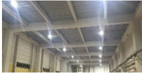
Installing LED based on green lease agreements
