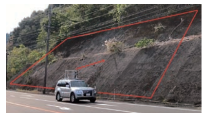
Image of slope surface
