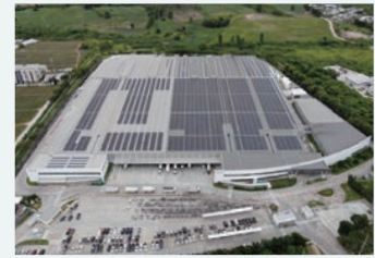
Roof of Ricoh Manufacturing (Thailand) Ltd. plant
