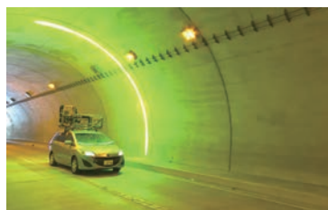
View of tunnel interior
