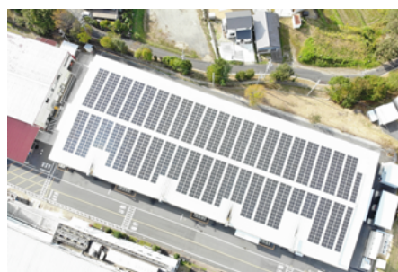
Roof of Ricoh Elemex Corporation plant
