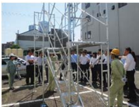
Demonstration of assembly at the temporary construction materials training
