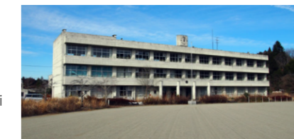
Closed school renovated for & HAUS
