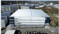
LOGIPORT Kobe Nishi Completed in Nov. 2021
