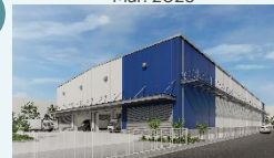
Matsudo Project Scheduled completion in Sep. 2024
