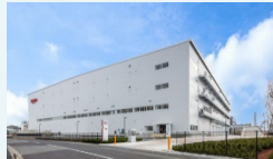
Matsudo Logistics Center Completed in Jan. 2022
