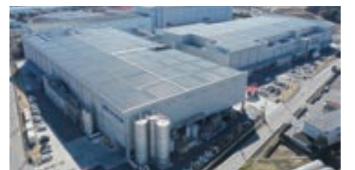
Solar panels installed on the roof of facilities in Kanto Yachiyo area
