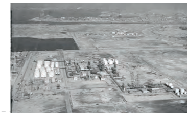
Nissan Petrochemicals Chiba Plant (1968)
