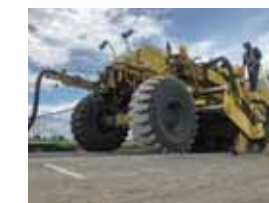
6 STABI-CEMENT RC construction method with road stabilizers using ICT technology
