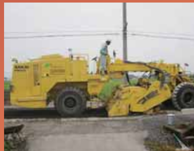
On-site base course recycling construction method STABI-CEMENT RC construction method
