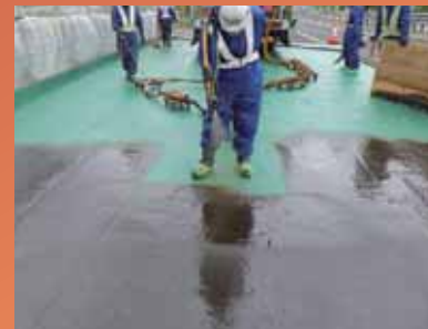
High-performance bridge deck slab waterproofing method HQ HIBRANE AU construction method
