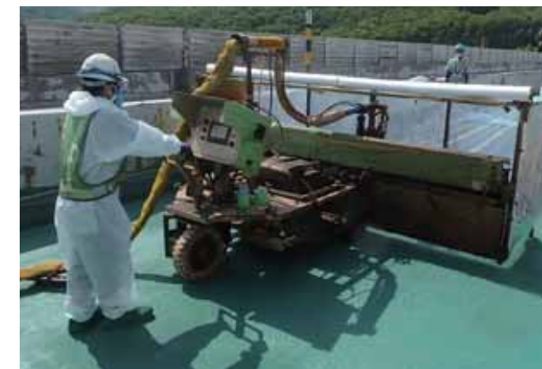
HQ HIBRANE AU construction method (construction with a binder spraying robot)
