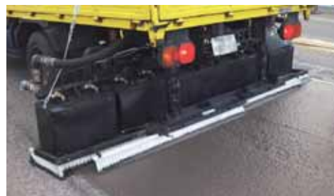
Dedicated vehicle applying and smoothing a thin layer of mixture
