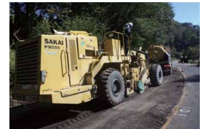
STABI-CEMENT RC construction method (mixing with a road stabilizer)
