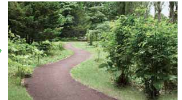
Example of constructed path
