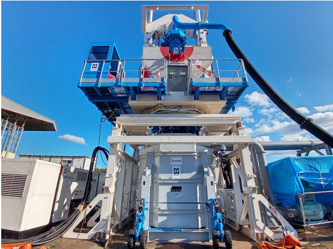
Exterior view of drilling equipment
