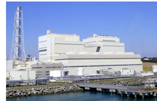
Haramachi Thermal Power Station
